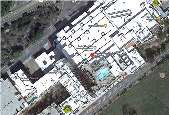
Aerial view of the facility with the cooling towers highlighted in yellow
